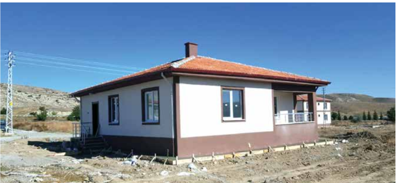
📍 Disaster housing (SHH) constructed in Çankırı
